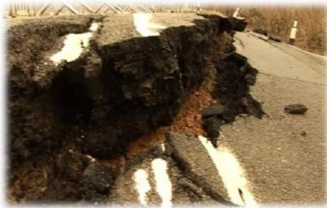
Oxford Road in Bagley Wood collapsed after the heavy rain in November 2012 saturated the ground. The road reopened a year later. Repairs cost £1 million.
