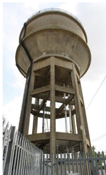
Figure 1 Picture of the water tower in Berinsfield
